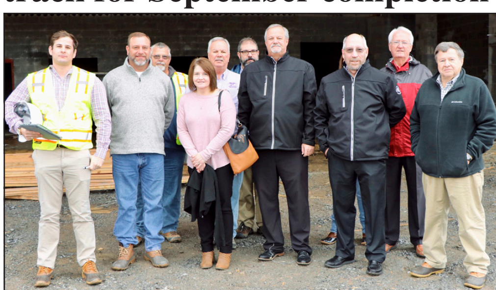
Stakeholders involved in the construction of the new Union County Double Gym held a tour of the unfinished facility last week.
